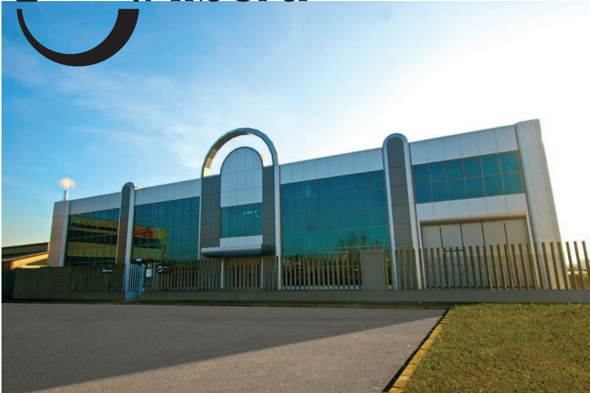
ALBERTI corporate facility located in Saronno (VA), Italy.
